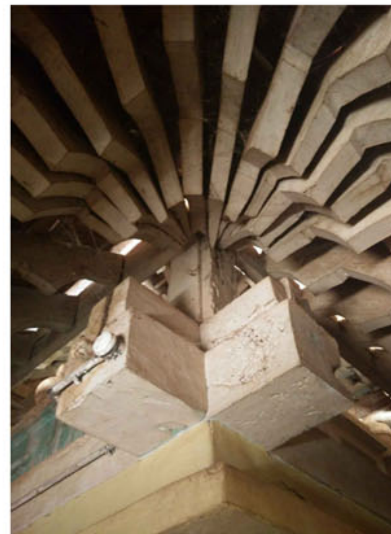
ANGULAR RAFTERS ON THE CRUCIFIX SHAPED CAPITAL - GARBHAGRIHA
